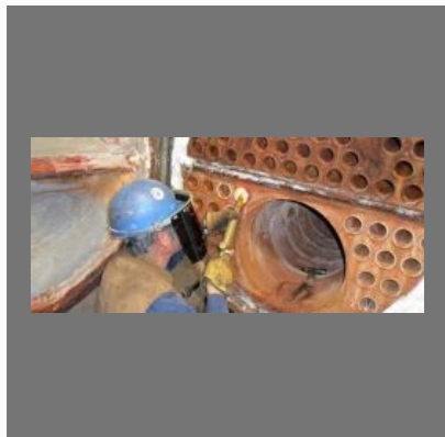
Steam Boiler Maintenance Services
