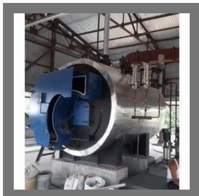
IBR Steam Boiler
