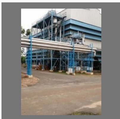
Pipe Line Works
