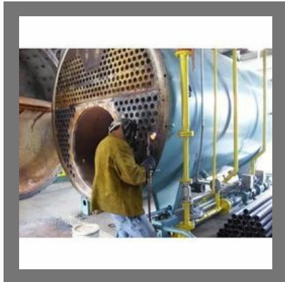
Steam Boiler Repair Service
